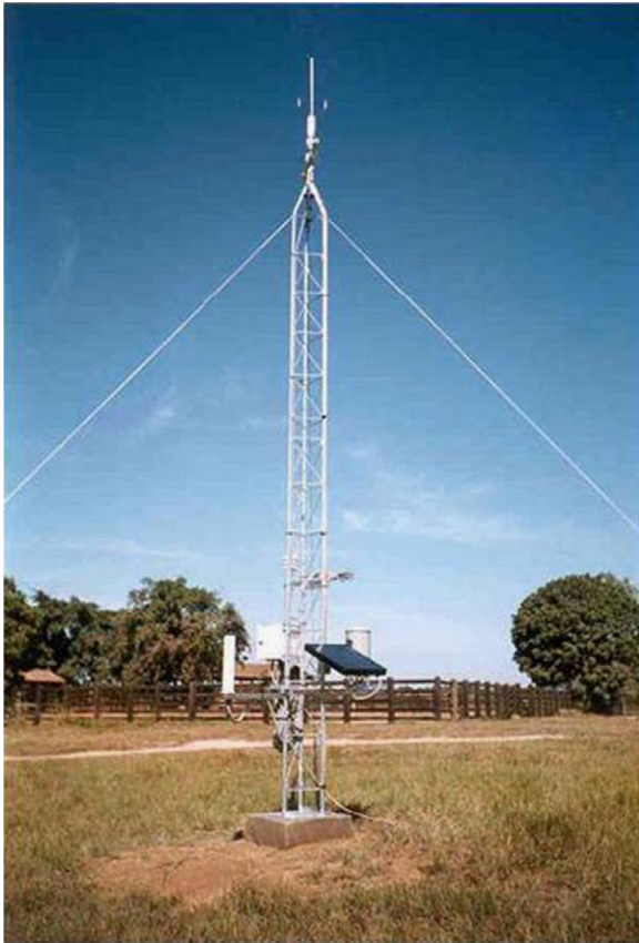
Fig. 2. Automatic station for environmental data collection. Courtesy: SINDA.
