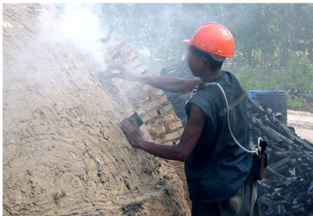
**Fig. 3** Occupational exposure of a kiln burner (a worker who supervises the burning process) and air sampling in the breathing zone (personal sampling)
