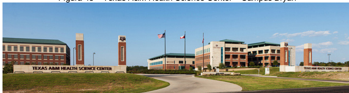
Figura 45 – Texas A&M Health Science Center – Campus Bryan
