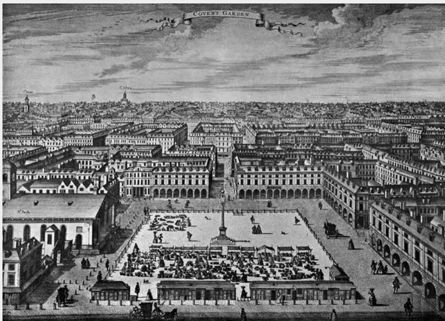
33. General view of Covent Garden looking north (cerca de 1720), gravura feita por Sutton Nicholls (1680-1740) e publicada pela primeira vez no London Described or the most noted Regular Buildings both Public and Private, with the Views of several squares in the Liberties of London and Westminster (1731). Praça do Covent Garden, em Londres, iniciada por Iñigo Jones (1573-1652), em 1631. Fonte: Wikimedia Commons contributors.
