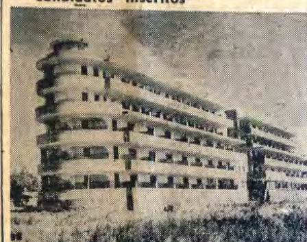
HOSPITAL SANTA TEREZINHA
