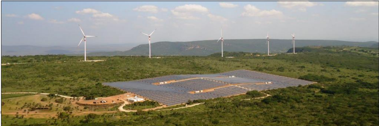
Figure 08. Hybrid power plant in Tacaratu/PE. Source: Enel Green Power Brazil, 2018. Adapted.
