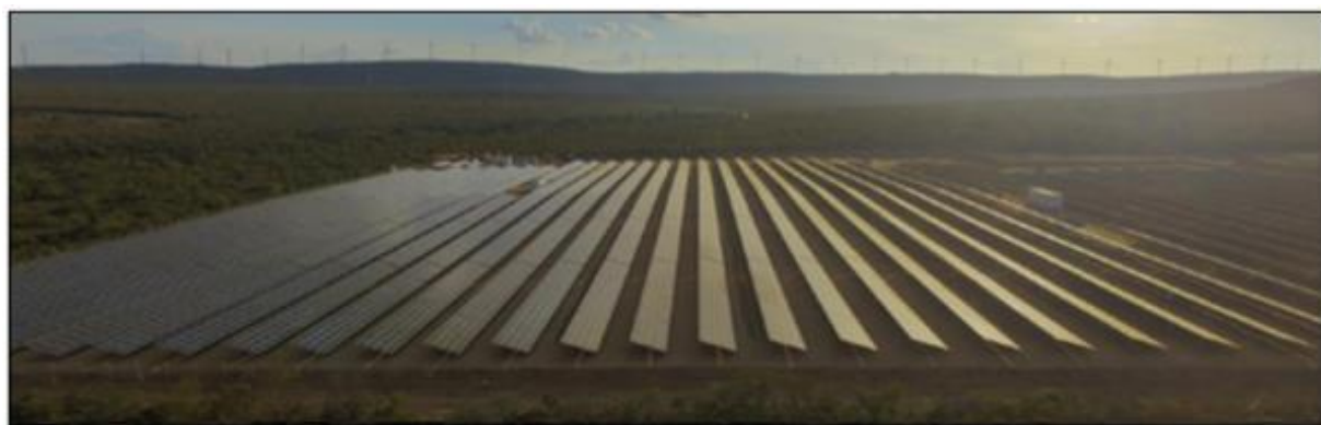
Figure 09. Hybrid power plant in Caetit  and Igaror /BA. Source: Renova Energia (2017). Adapted.
