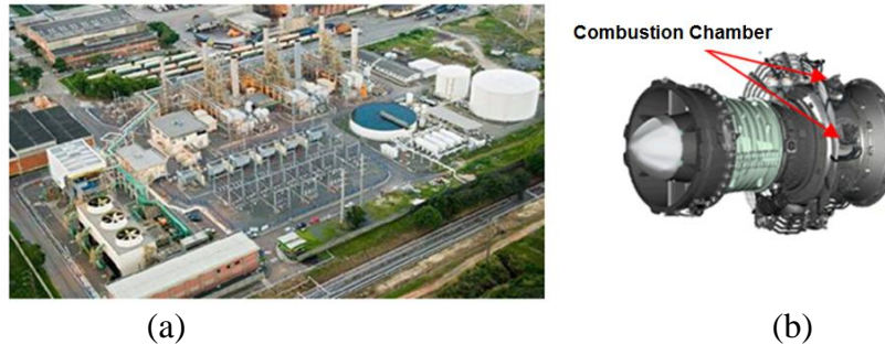
Figure 9 – (a) TPP and (b) Gas turbine RB211-G62 DF ((Fontes and Pereira, 2016), (Fontes and Budman, 2017), (Rolls-Royce, 2010))
