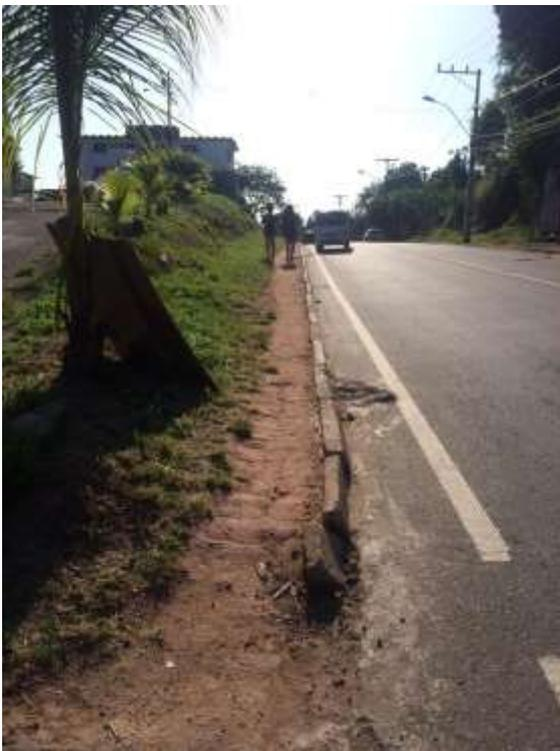
**Figura 37:** calçada sem pavimentação
