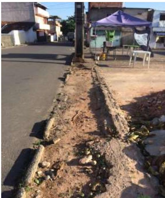
**Figura 33:** inexistência de calçada
