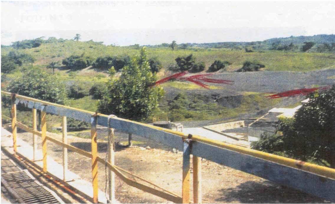
Photo 6.2 - Slag bus with red signs indicating area to be worked on. Source: GONÇALVES (2001).
