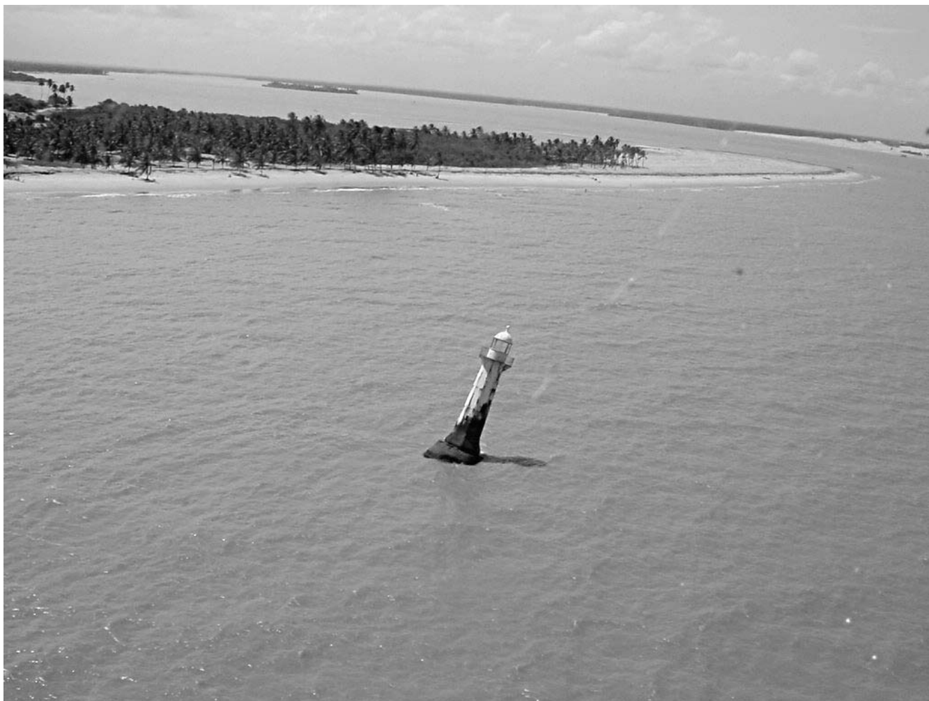
Figure 3. Right bank of the São Francisco River mouth, now without the village of Cabeço. The lighthouse can be seen already approximately 200 m from the shoreline (2002).
