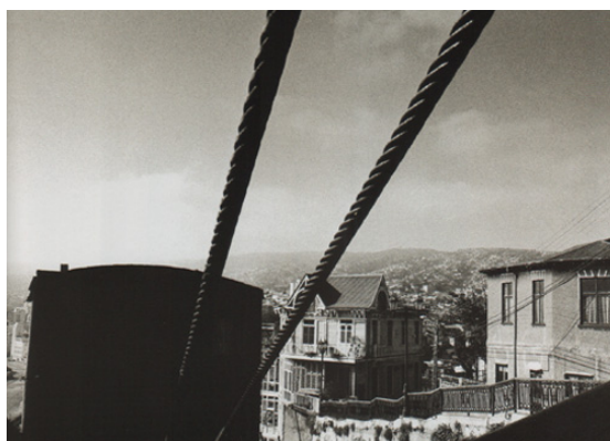
fig. 48. Eduardo Couve, “ Main and Auxiliary Cables ”, Ascensor Artillería, Cerro Artillería, 2002. (COUVE, 2003, p. 66)
